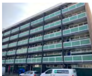
REPEATED MODULAR FACADE
