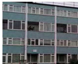
PRE-FABRICATED PANELS
