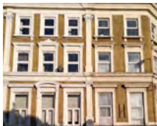
YELLOW STOCK BRICK WITH STUCCO
