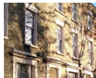
WHITE LINTELS & ARCHITRAVES
