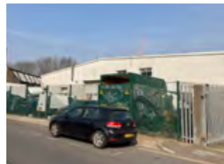
CORRUGATE METAL SHEDS
