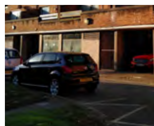
GROUND FLOOR GARAGE SPACE
